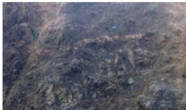
Figure 5: Weathered and Disintegrated Rock Mass Quality at Asprovalta – Strymona’s Part of Egnatia Highway at Northern Greece
