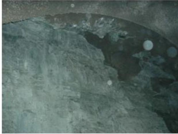
**Figure 6: Chloritic Schist Rock Mass during Tunneling of Symbol Mountain at Strymonas-Kavala's Part of Egnatia Highway at Northern Greece**
